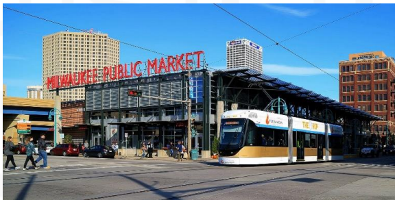
The Hop streetcar opened its first phase in Fall 2018 and is exceeding ridership projections, while also triggering several new development projects. Route expansions are currently being designed.
