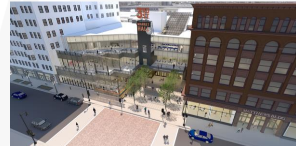
The Shops of Grand Avenue is undergoing a $90 million redevelopment into The Avenue that will include offices – anchored by GRAEF, residential units, retail, and the 3 rd Street Market Hall
