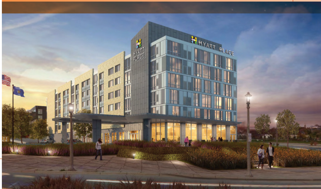
HYATT PLACE – The 150-room hotel overlooking the new Bucks arena and Milwaukee’s scenic skyline includes a bar serving breakfast that will later transition into a full-service bar and restaurant.
