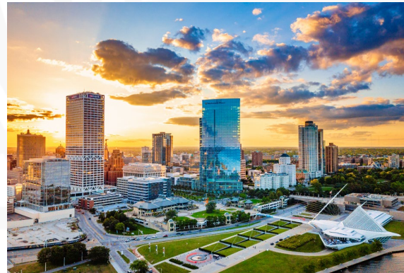
833 East & Northwestern Mutual's headquarters are two of several new developments near the lakefront in the Central Business District
