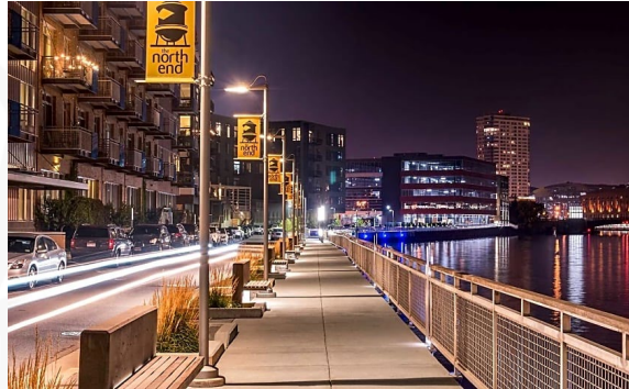
Thousands of new apartments have led to a 26.5% increase in the downtown residential population since 2010, bringing it to more than 32,000 residents
