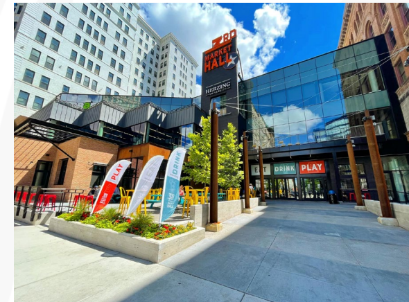
The Shops of Grand Avenue underwent a $100 million redevelopment into The Avenue that will include offices – anchored by GRAEF, residential units, retail, and the 3 rd Street Market Hall
